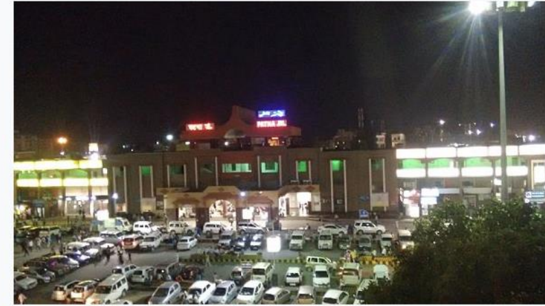
The main entrance of the station
